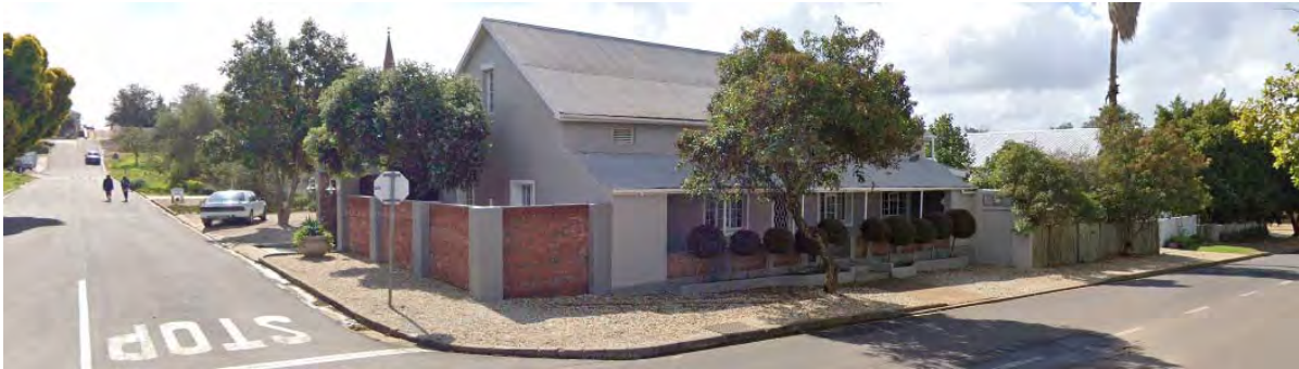
Façade facing Piet Retief Street
