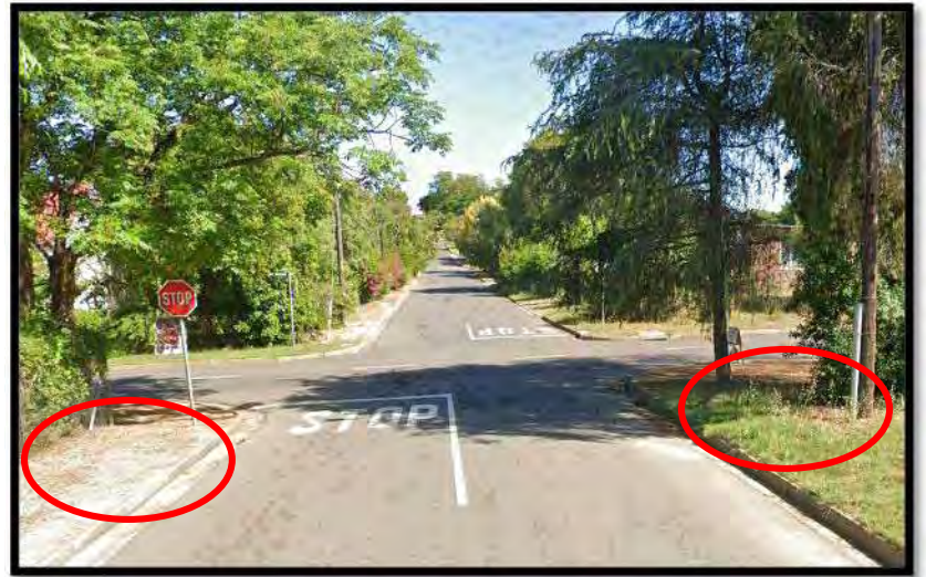
Figure 2: Existing sidewalk encroachment on Royal Street
