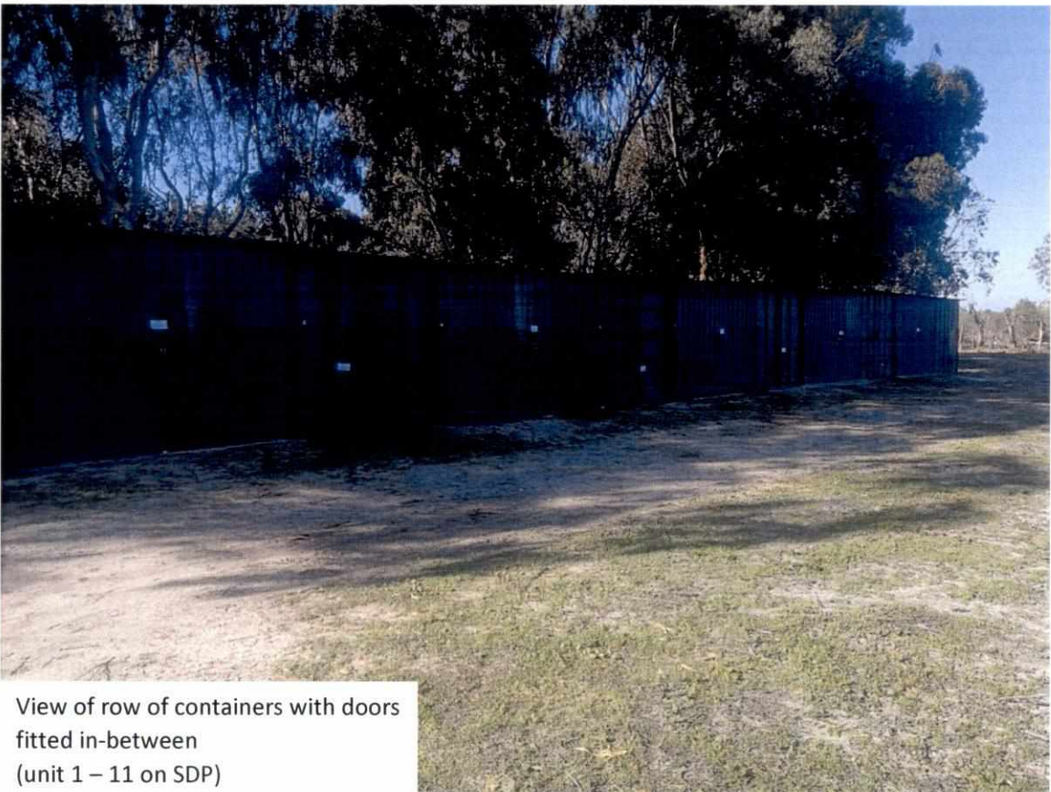
View of row of containers with doors fitted in-between (unit 1 – 11 on SDP)
