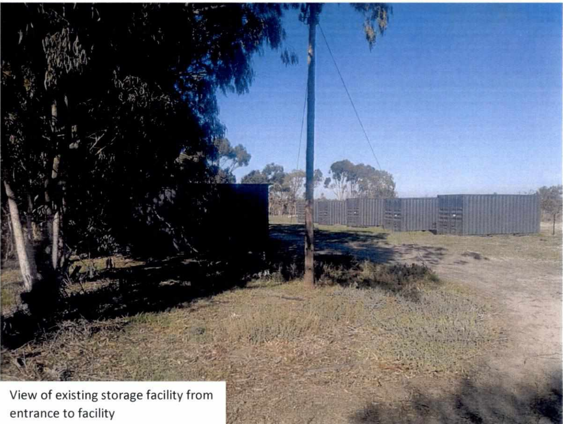
View of existing storage facility from entrance to Farm 39/554
